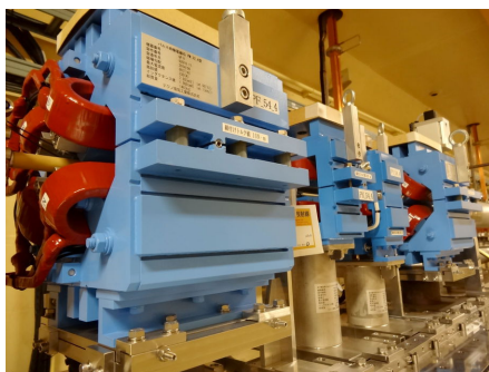
Figure 2: Example of pulsed magnets installed in the linac.
