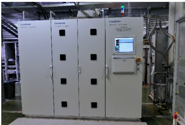
Figure 4: 130 kW 500 MHz amplifier.
