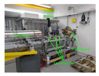
Figure 3: Most of the beam line elements in front of the undulator are installed and aligned. The switchyard magnet support frame was modified and will be aligned shortly and after that the missing bellows and beam tubes to connect the beam line to the undulator vacuum chamber can be installed.
