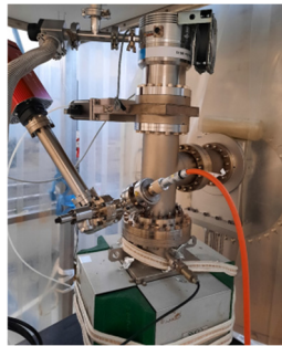
Figure 2: High speed pumping group (~60 L/h) connected to the beam gate valve of the cavity string.
