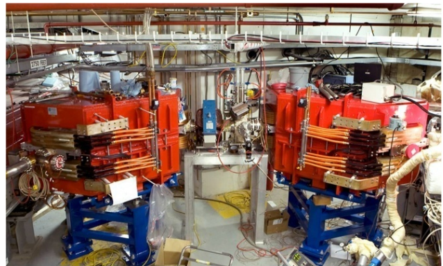
Figure 6: Dipoles installed in the Booster tunnel.
