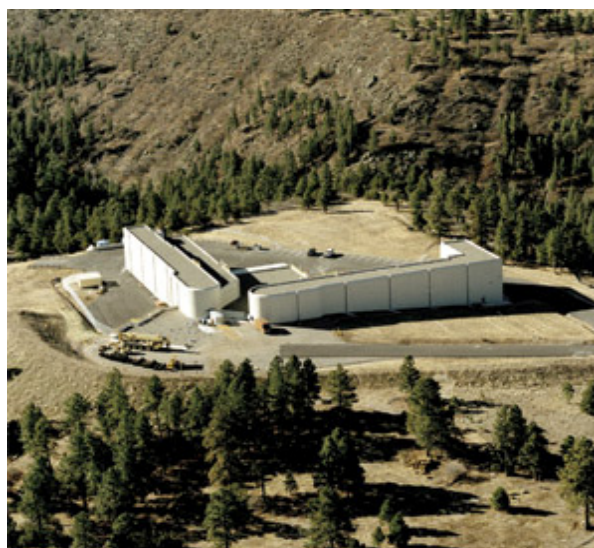
Figure 1: Aerial view of the Dual Axis Radiographic Hydrodynamic Test (DARHT) facility at the Los Alamos National Laboratory.
