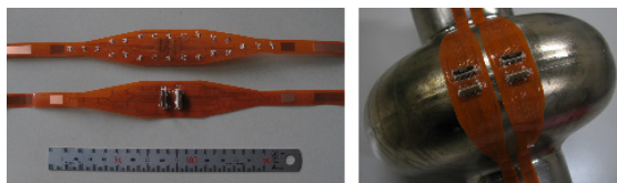
Figure 7: Experimental sensor strips resistors on flexible polyimide film contact with surface of Niobium cavity.
