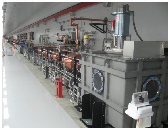
Figure 10: Installation of injector section (by MHI).
