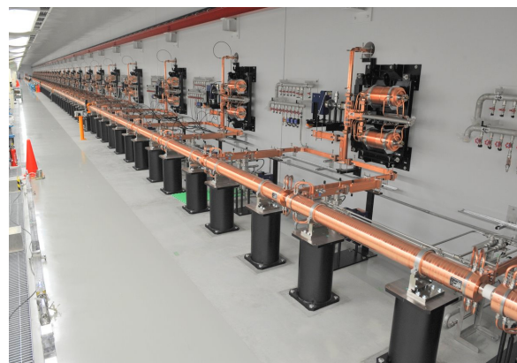
Figure 9: Installation of C-band section (by RIKEN).
