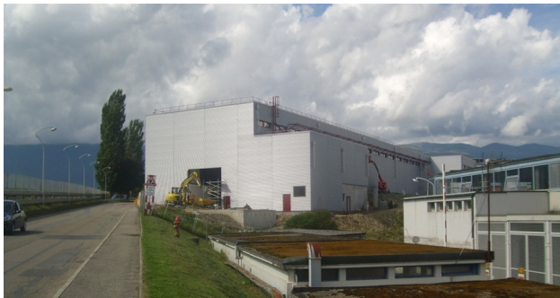
Figure 5: Linac4 building completed.
