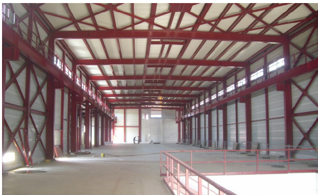
Figure 6: Surface equipment hall.
