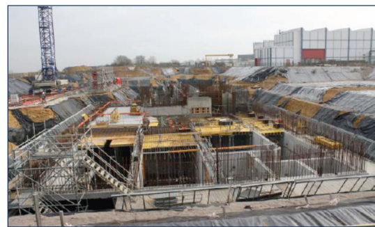
Figure 9: View of the construction site (May 2012)
