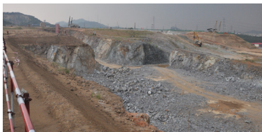
Figure 1: Civil construction status of the linac tunnel.
