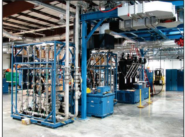
Figure 3: The 402.5 MHz klystron and its cooling cart have already been installed along with a portion of the waveguide system. A trio of 550 kW, 805 MHz klystrons is visible in the background, where a separate klystron testing capability is being established.
