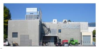
Figure 1: New HIE-ISOLDE service buildings housing cryogenics, cooling & ventilation and RF systems.
