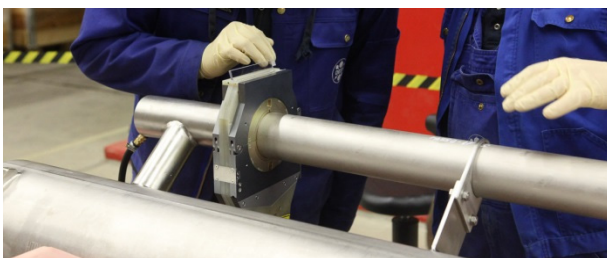
Figure 6: Welding a seamless pipe
