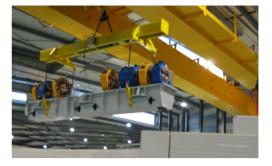
Figure 6: Moving the first girder into the tunnel.
