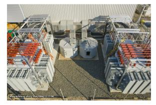
Figure 6: The New AGS MMPS Transformers.
