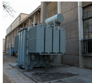
Figure 5: Choke construction.
