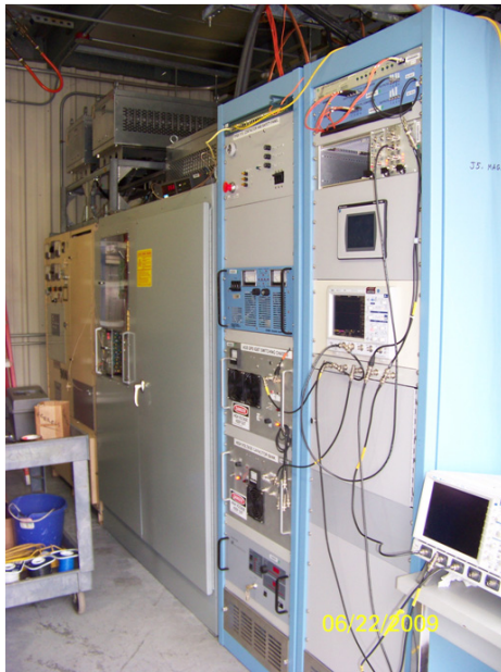
Figure 7: A complete tune jump power supply.
