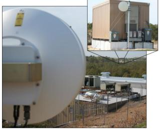
Figure 7: The microwave link transmitter for the Yellow ring, above the pickup in sector 2, is shown in the foreground. The receiver and dedicated electronics trailer, above the kicker in sector 11, are shown in the distance and the inset.
