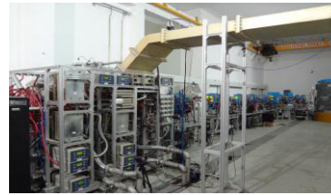
Figure 19: CPHS linac under beam tuning.
