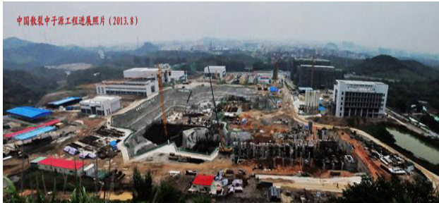
Figure 2: Civil construction status of CSNS project.
