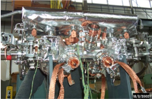
Figure 8: Cold mass assembling in the workshop.
