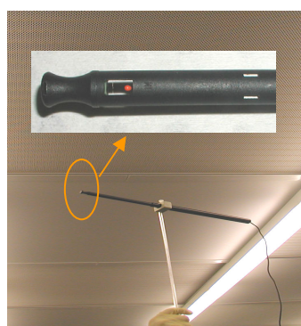
Picture 2: Detailed view on set up for air velocity measurements
