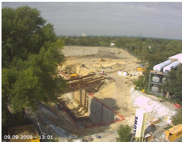
Figure 2: Construction site of the XFEL injector.
