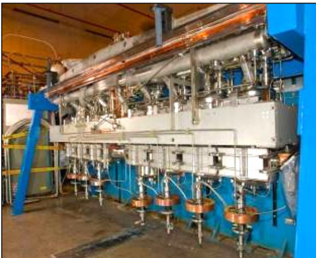
Figure 9: Dressed string suspended from cryomodule lid.
