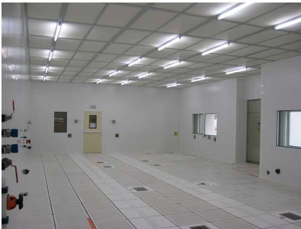
Figure 5: the new large ISO 4 clean room being built at CEA Saclay.
