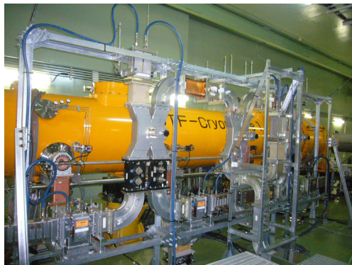
Figure 4: Installation of the cryomodule in the STF tunnel.
