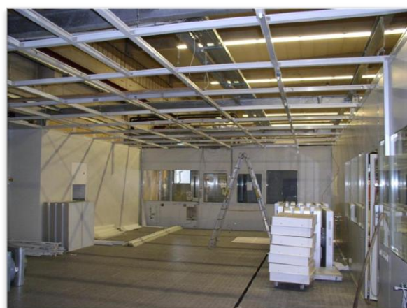
Figure 1: Main clean room area (ISO 4/5) before installation of FFU's.
