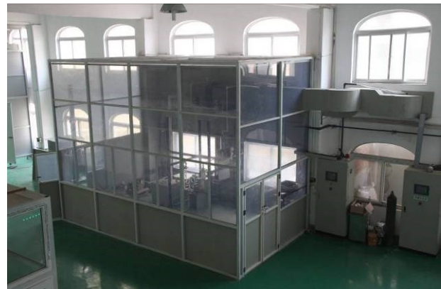
Figure 2: BCP Facility at Daxing base of IHEP.
