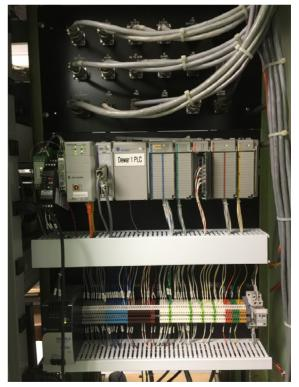
Figure 3: Dewar control PLC and I/O.
