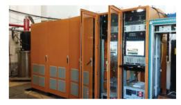
Figure 10: 1.3 GHz 5 MW klystron and Marx modulator.
