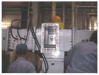
Figure 4: Installation of the asymmetric power divider.
