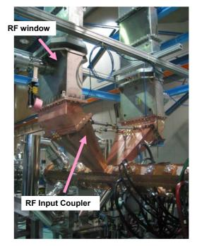
Figure 2: RF window, RF input coupler
