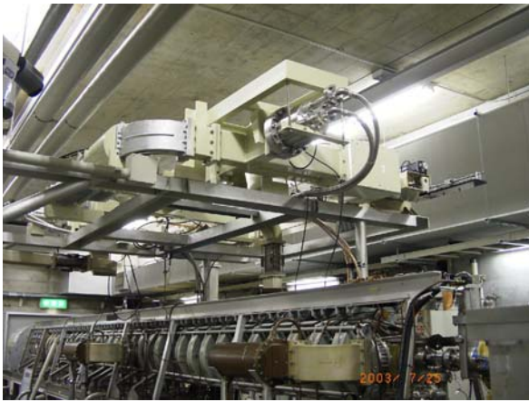
Fig. 2. Wave guide system assembled above the linac.
