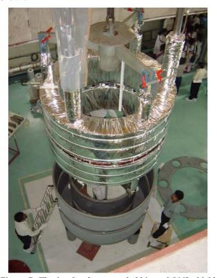
Figure 7: The insulated cryostat bobbin and LN2 shield assembly is being installed within the iron vacuum chamber (Coil Tank).
