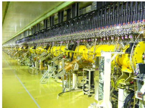
Figure 5: DTL1,2,3 in the tunnel
