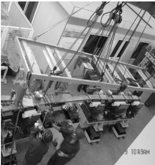
Figure 8: Suspend and install the chambers
