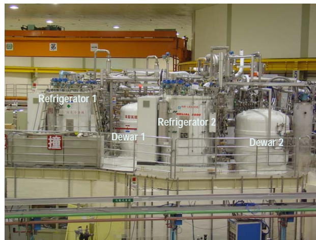
Figure 2: The infrastructure of installed cryogenic system in the experimental hall.
