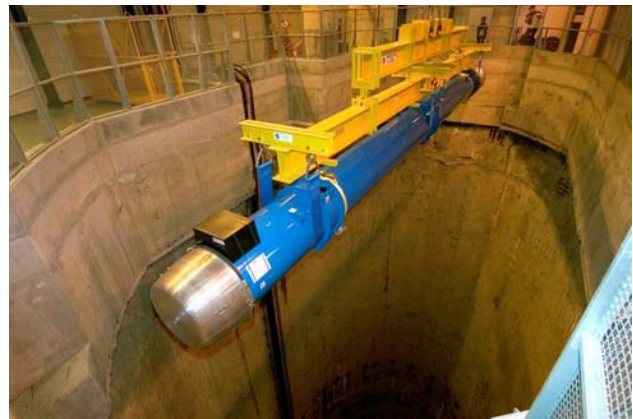
Figure 4: Lowering of a dipole.
