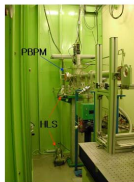
Figure 1 : Installation of Photon Beam Position with Hydraulic Level System. HLS are installed on the floor and support.
