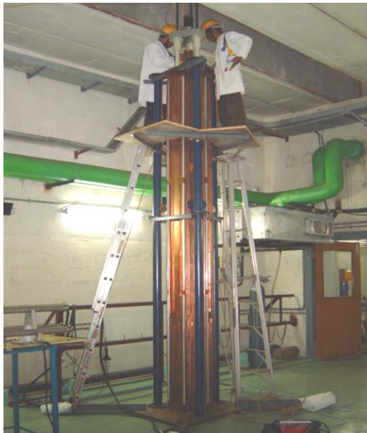
Figure 19: One of the six RF resonators being assembled at VECC.
