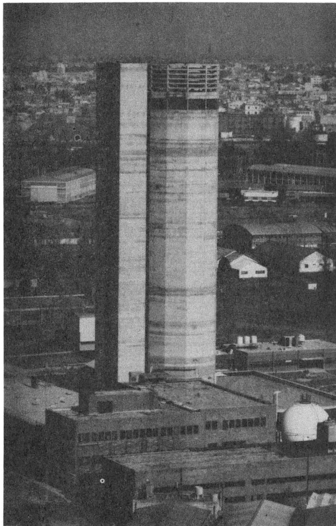
Fig. 5. External view of the Buenos Aires Tandem Accelerator Facility under construction.
