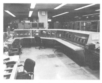
Fig. 1. Central operator console.
