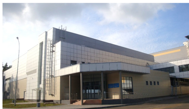
Figure 1: Building of SHE Factory.
