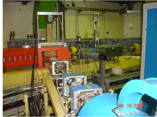
Figure 4: A GigE Vision camera installed at exit of 50 MeV linear accelerator for test.
