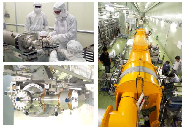
Figure 3: Attachment of an input coupler in a clean room, (Left, top). An assembled cavity mounted under the 2 K gas-return pipe, (Left, bottom). A 6-m long cryomodule installed in the STF tunnel, (Right).
