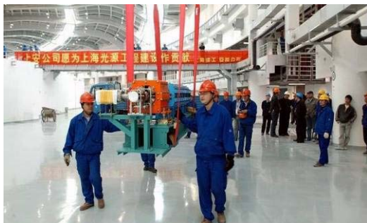
Figure 8: The first booster unit started installation
