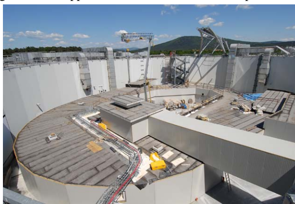
Figure 1: Booster building during construction, May 2007.
