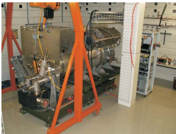
Figure 3: The high voltage high gradient test facility at PSI: the 500 kV pulser is installed and being commissioned.
