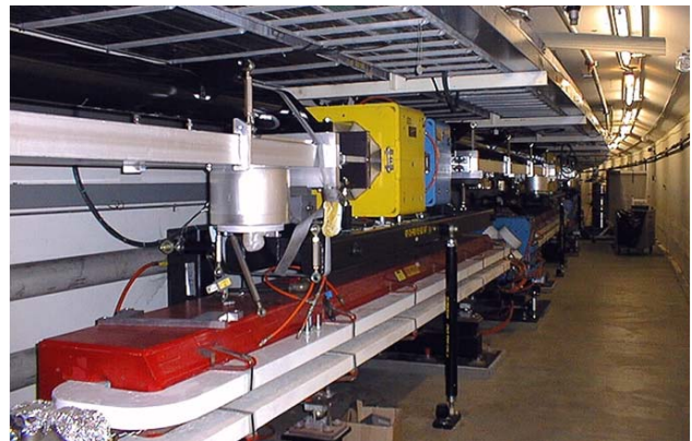
Figure 1. Tunnel layout of the two beam lines. The LER is above the HER.
