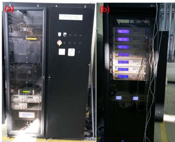
Figure 7: Control system of cryomodules for (a) PLC rack and (b) temperature monitors.
